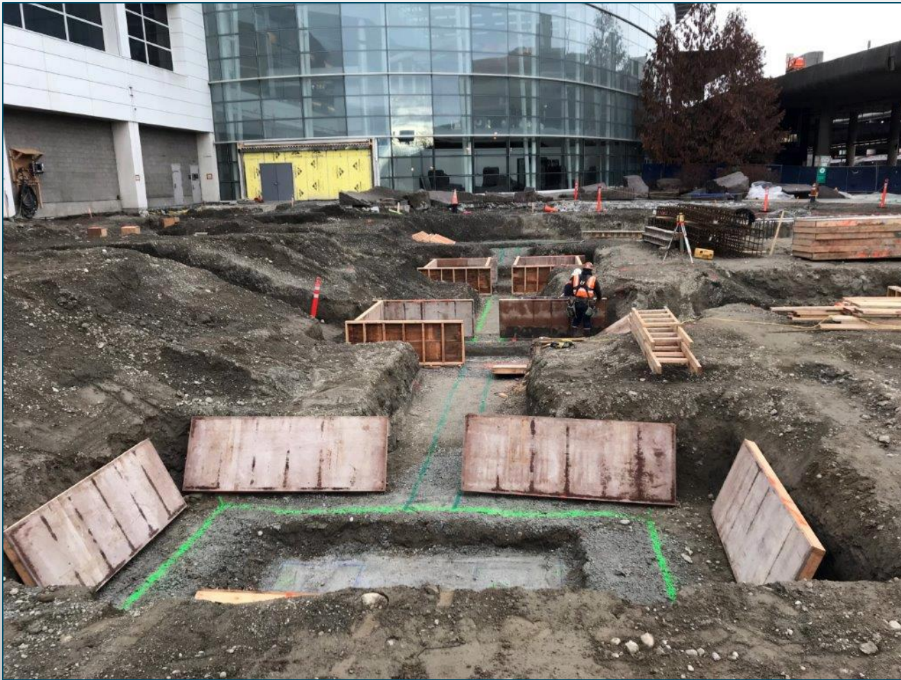
Landside Construction Progress
