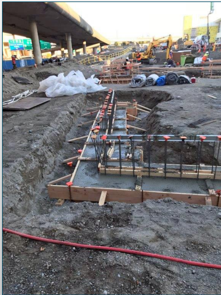
Landside Construction Progress
