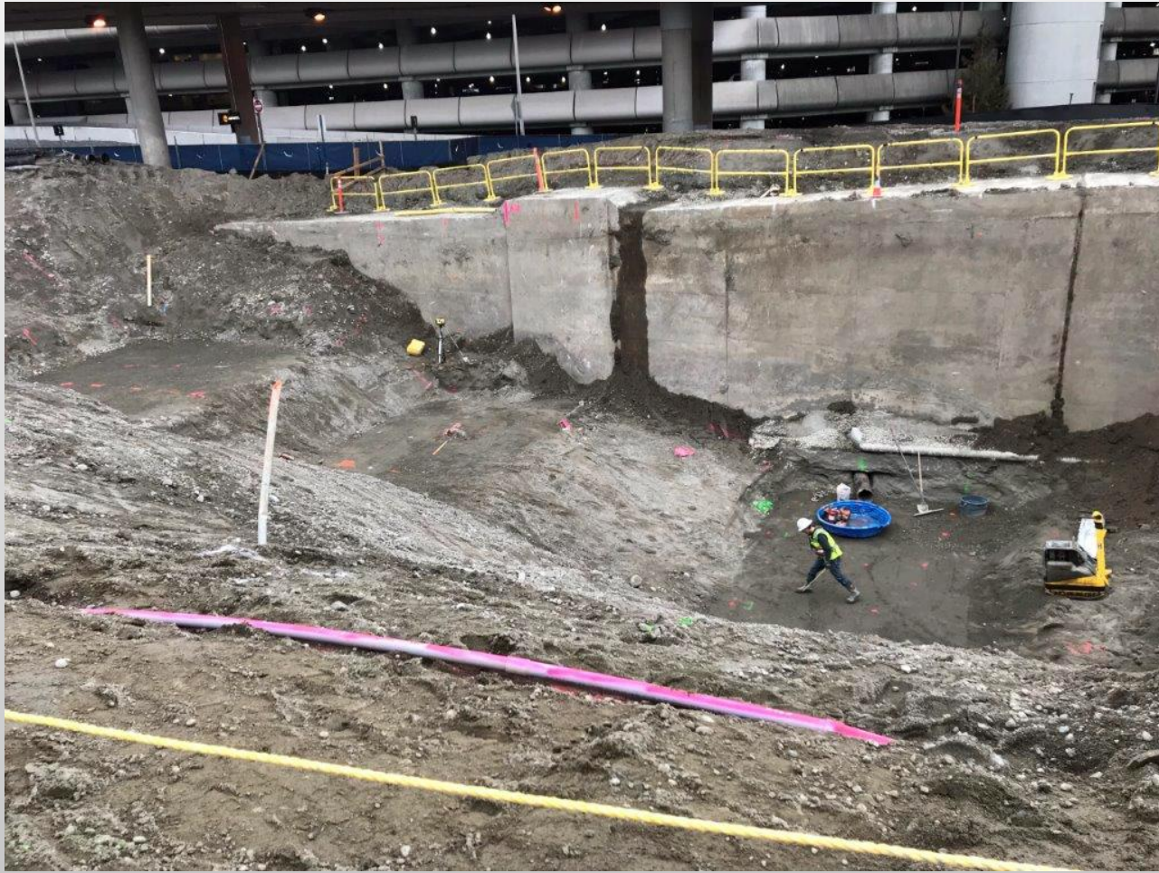
Landside Construction Progress
